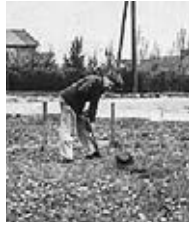
2 nd April 1953 Ejnar Pedersen digs for foundations of PP Møbler
