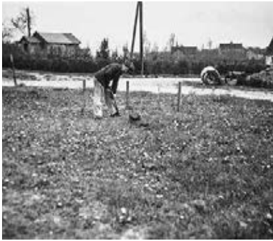
2 nd April 1953 Ejnar Pedersen digs the foundations of PP Møbler
